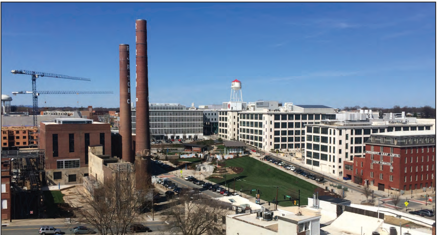
The Innovation Quarter North District (photo courtesy of IQ)
